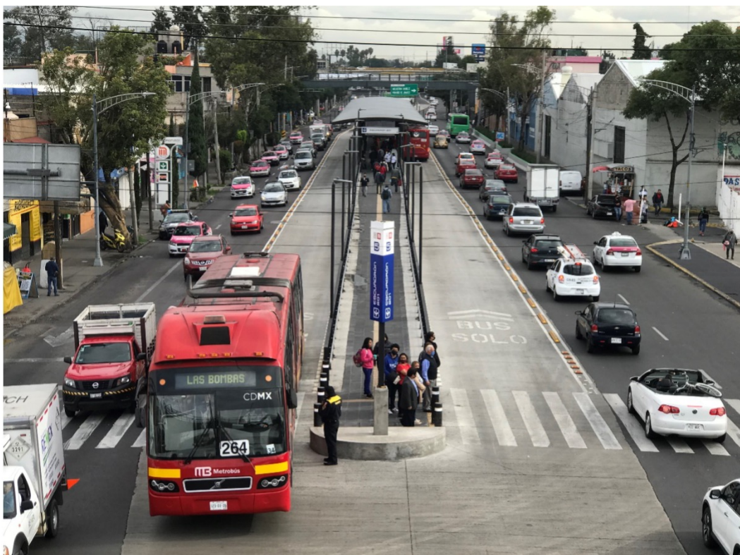
Figure 11: Line 5, Station Escuadrón 201 (Metrobús, 2024)
