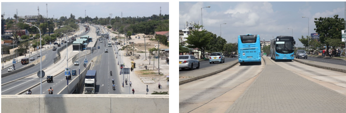
Figure 3: BRT in Dar Es Salaam. Source: Dar Rapid Transit Agency, 2024
