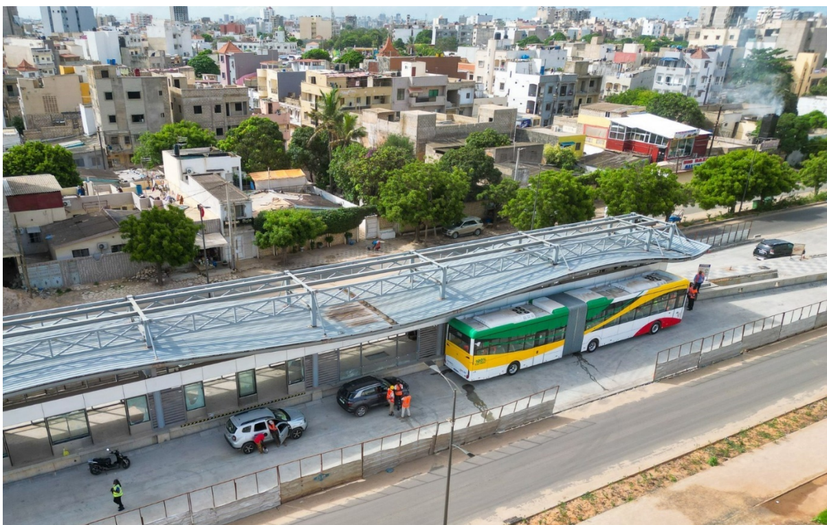
Figure 4: Dakar's BRT connects downtown Dakar and the suburb of Guediawaye. Photo: CETUD - Conseil Exécutif des Transports
