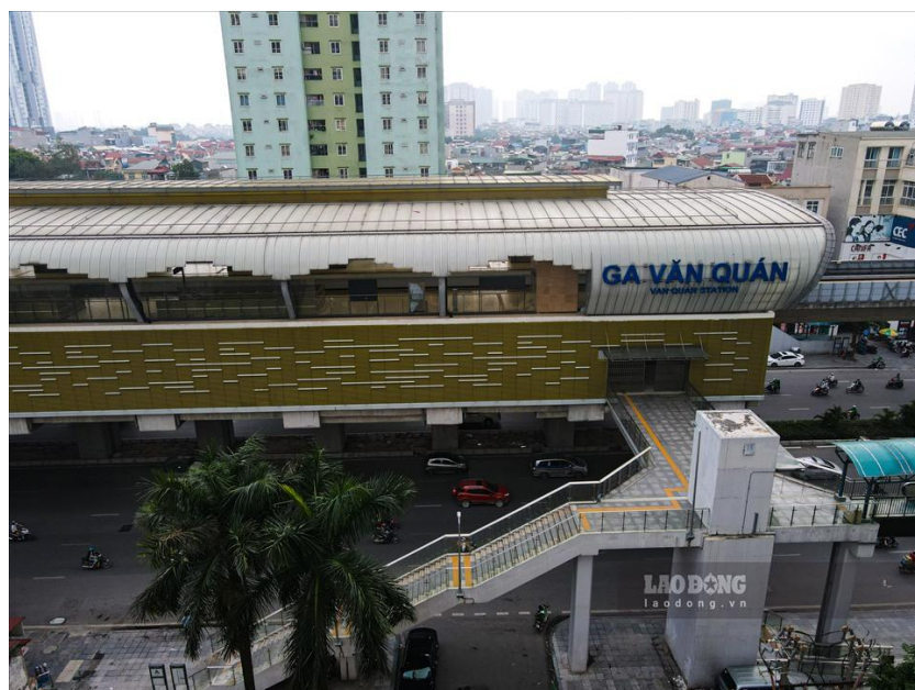
Figure 2: Van Quan metro station
