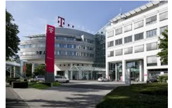
Office buildings, parking space
