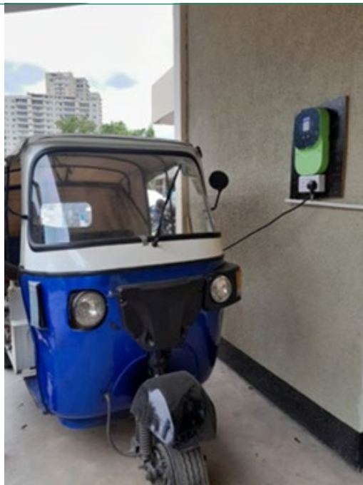
Location of the chargers deployed by TRI for DART, at or near BRT stations
