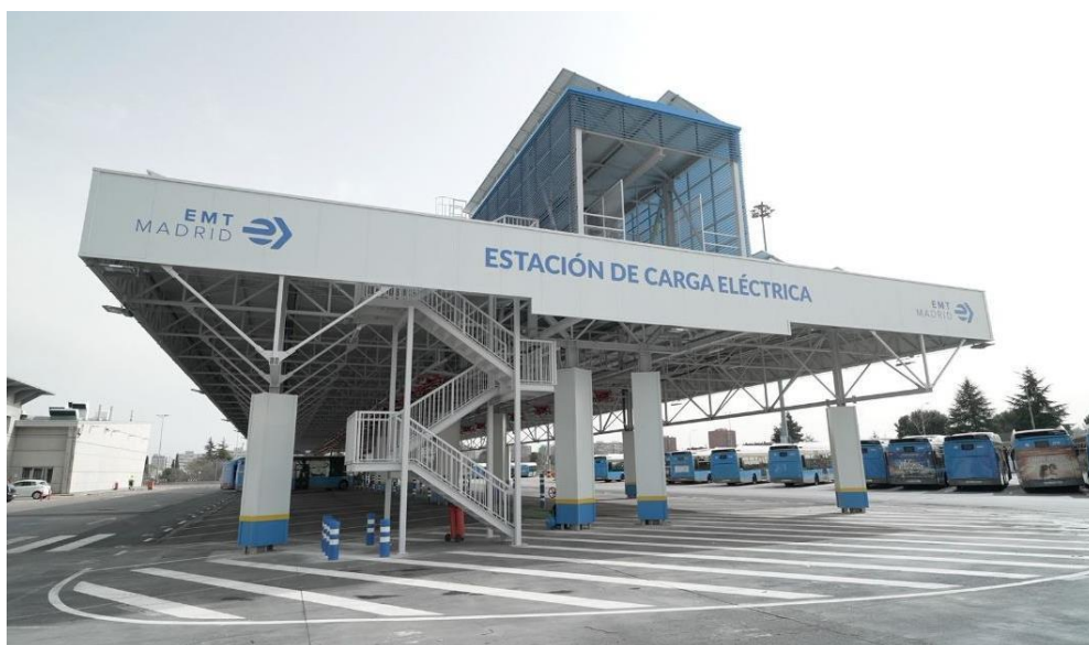
Figure 1: Phase II of the inverted pantographs in Carabanchel bus depot
