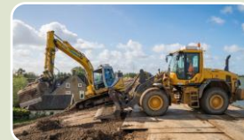
Sterke Lekdijk H2 construction equipment
